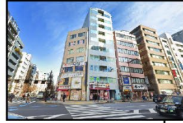
Distribution Hub Tokyo (Japan)
