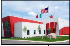
Distribution Hub Shakopee, MN (USA)
