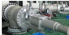
The Company delivers a 600-mm moisture separation heater escape valve to the AP1000 Sanmen No. 1 Nuclear Power Plant in China.
