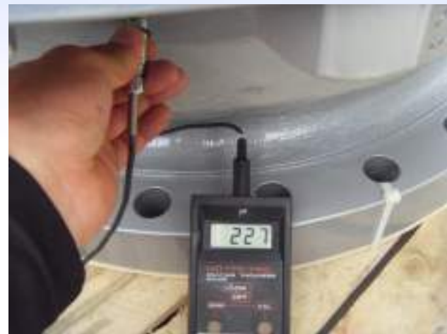
Paint Thickness TEST
