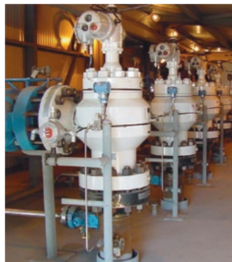
CC80 choke with electric actuation
