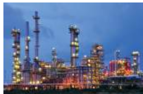
Installed on petrochemical plants all over the world
