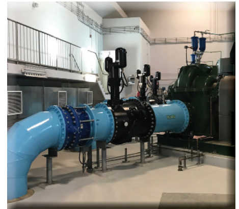
American-BFV® Butterfly Valves, Tilted Disc® Check Valves, Combination Air Valves & Silent Check Valves Ontario, Canada
