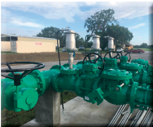
Cam-Centric® Plug Valves, Swing Check Valves & Combination Air Valves Winter Haven, FL
