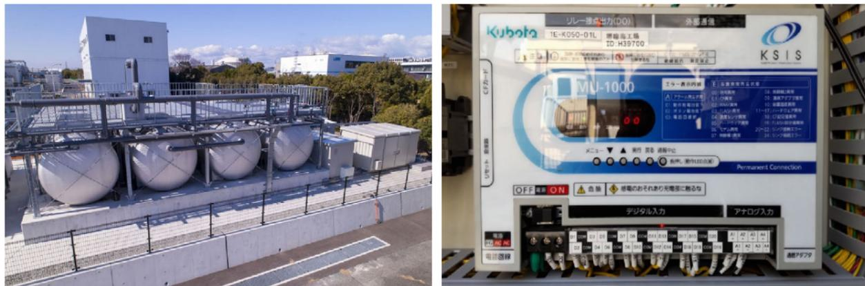
At the Kubota Sakai Rinkai Plant, we expanded our installation of submerged type FRP *johkasou*, decentralized wastewater treatment plants. These are able to handle high-level treatment of household wastewater and can process up to 110 m<sup>3</sup> of wastewater per day. Furthermore, as a BCP measure, we have raised the concrete foundations of the wastewater treatment facility. We introduced a water management solution using IoT, "KSI S," to realize proper management of plant wastewater.
