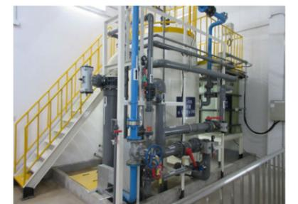
At Kubota Agricultural Machinery (Suzhou) Co., Ltd. (China), we installed recycling treatment equipment for reusing wastewater from processes throughout the entire plant, and this has realized zero emissions of process wastewater.
