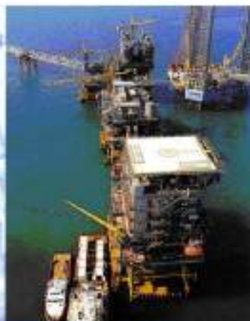
Offshore gas production platform
