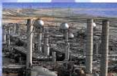
Onshore gas production facility
