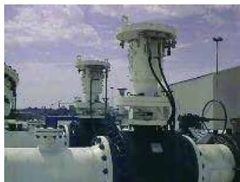
Rotary vane double-acting actuator
