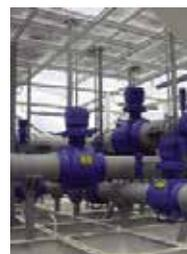
Gear operators with reach rods in a subsea manifold
