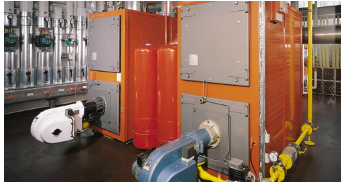
Gas inlet pressure monitoring on high-performance boilers
