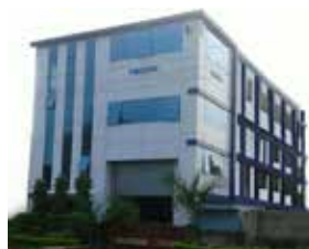
Tecnik Fluid Controls Pvt. Ltd. Mumbai, India
