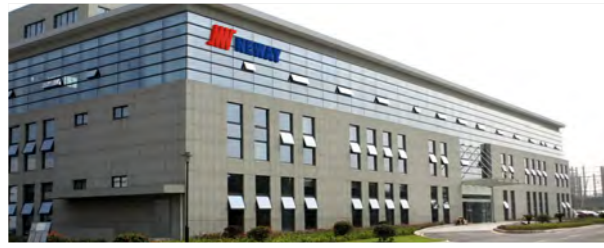
NEWAY Head Office Founded in 2014 Total area: 2,295sqm Office area: 6,885sqm
