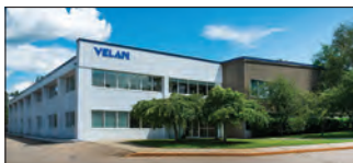
Williston, VT, U.S.A. Velan Valve Corp., Plant 3
