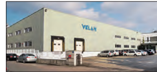
Ansan City, South Korea Velan Ltd., Plant 2
