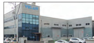
Ansan City, South Korea Velan Ltd., Plant 3
