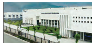
Suzhou, China Velan Valve (Suzhou) Co., Ltd.
