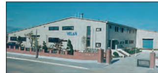
Ansan City, South Korea Velan Ltd., Plant 1
