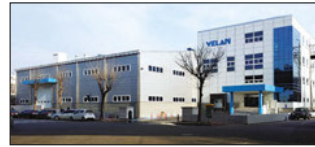
Ansan City, South Korea Velan Ltd., Plant 1
