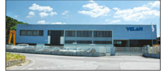
Lucca, Italy Velan ABV S.r.l., Plant 1
