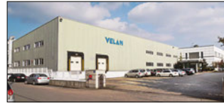
Ansan City, South Korea Velan Ltd., Plant 2
