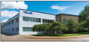
Williston, VT, U.S.A. Velan Valve Corp., Plant 3
