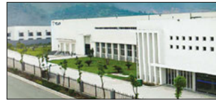
Suzhou, China Velan Valve (Suzhou) Co., Ltd.
