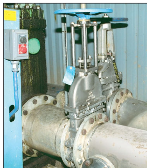
Filter isolation installation.
