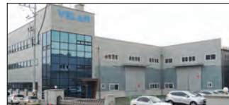
Ansan City, South Korea Velan Ltd., Plant 3
