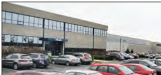
Montreal, Canada Velan Inc., Plant 5
