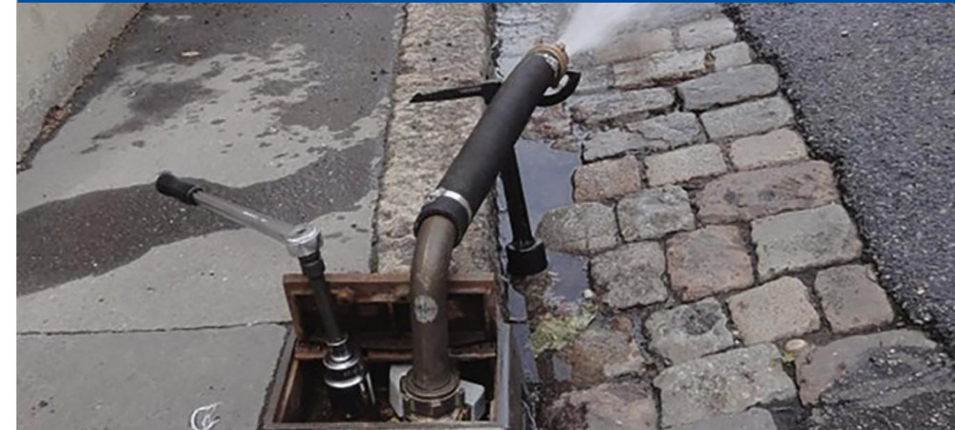
*The metering tool for underground water hydrants*
