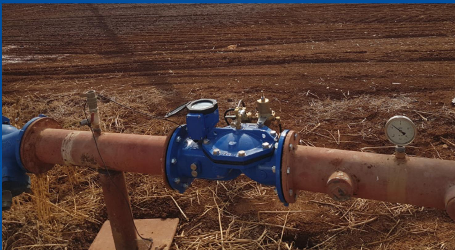
The ULTRAF combines the highest level of pressure and flow control valve with an accurate and reliable Ultrasonic water meter in one compact design. ULTRAF PRO combines state of the art technologies from different fields, such as advanced hydraulics, accurate sensing and modern communications.
