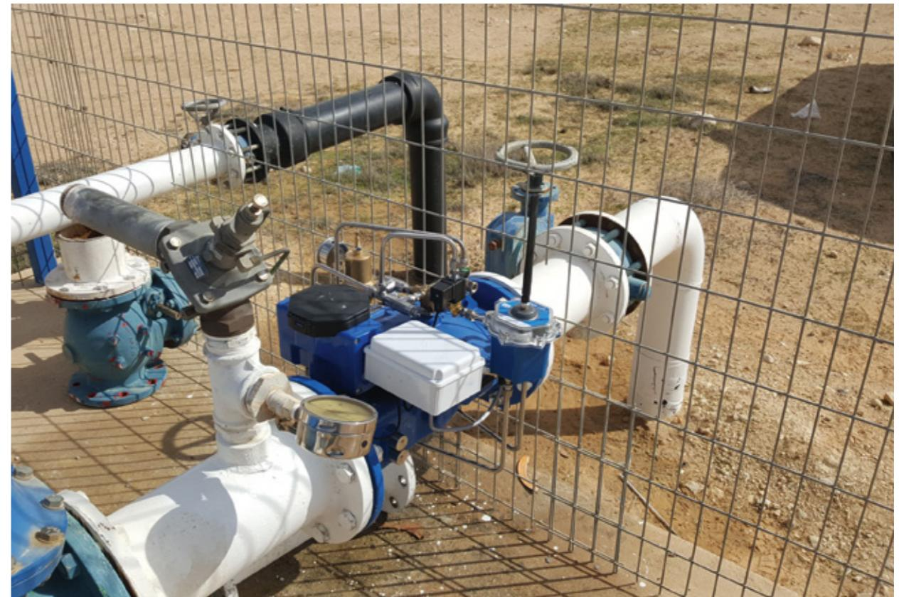
Apollo smart Data logger along with the Ultraf Ultrasonic Hydrometer on the main water line inlet of Tlalim Village
